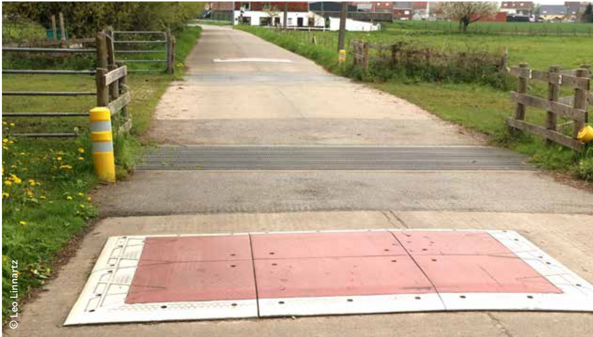
Fig 6.3 Fragmentation can be mitigated by connecting two grazing areas across a road. Reducing traffic speed, e.g. by using speed bumps, is highly advised.
